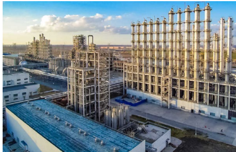
Daqo polysilicon production facility. Source: Daqo New Energy Corp
